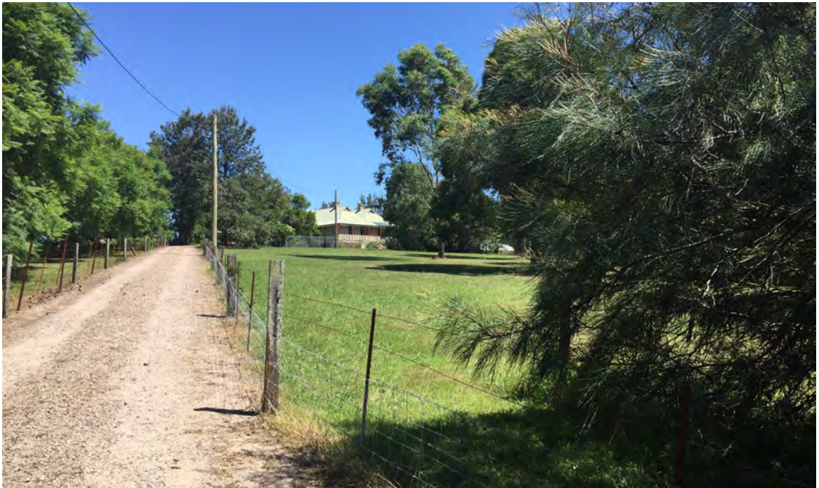
Photo 4 – View of entrance to #394 Hinton Road
